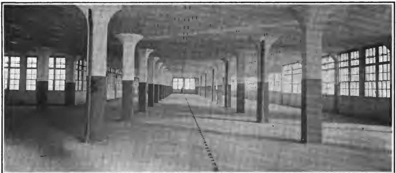
Ground floor of the new storehouse and unit assembly building. This floor is now being used for the reception of raw material. The second floor of this building, exactly similar in aspect, is used for finished stock and the third and fourth for the assembly of units such as motors, transmissions, rear axles, carburetors, steering gears, pumps and clutches.
